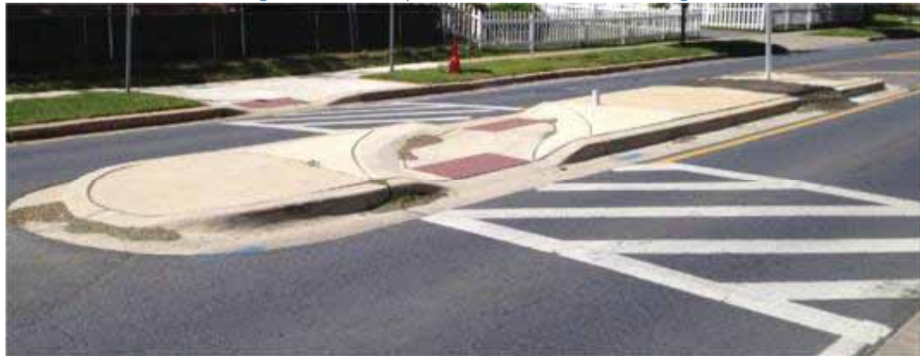
Figure 23-12: Example of an Offset Crosswalk and Pedestrian Island
