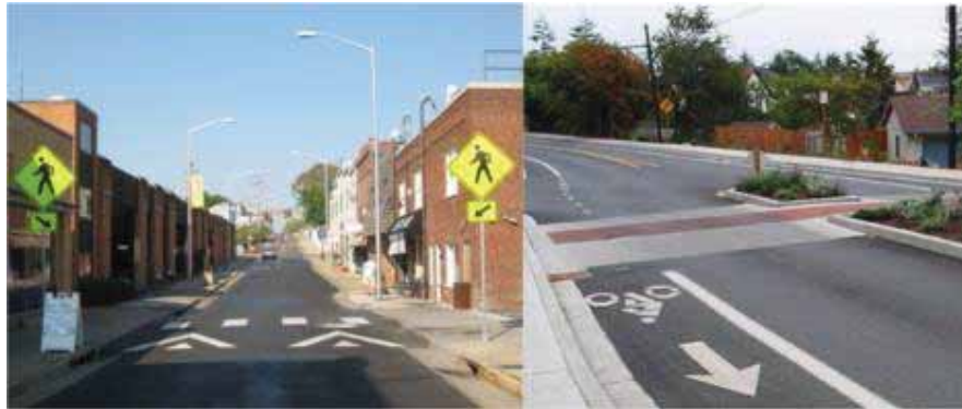
Figure 23-20: Examples of Raised Pedestrian Crossing
